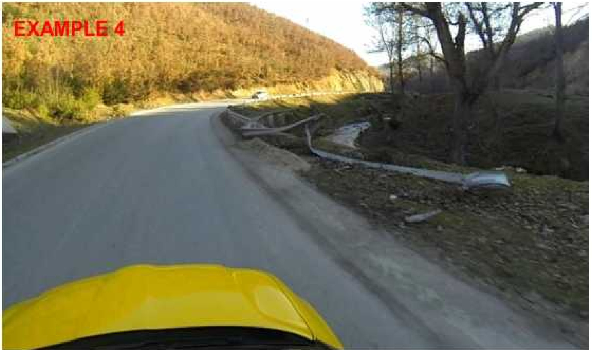
Example 4 – Unrepaired safety barriers deformed from previous accidents are commonly present on Albanian roads.
